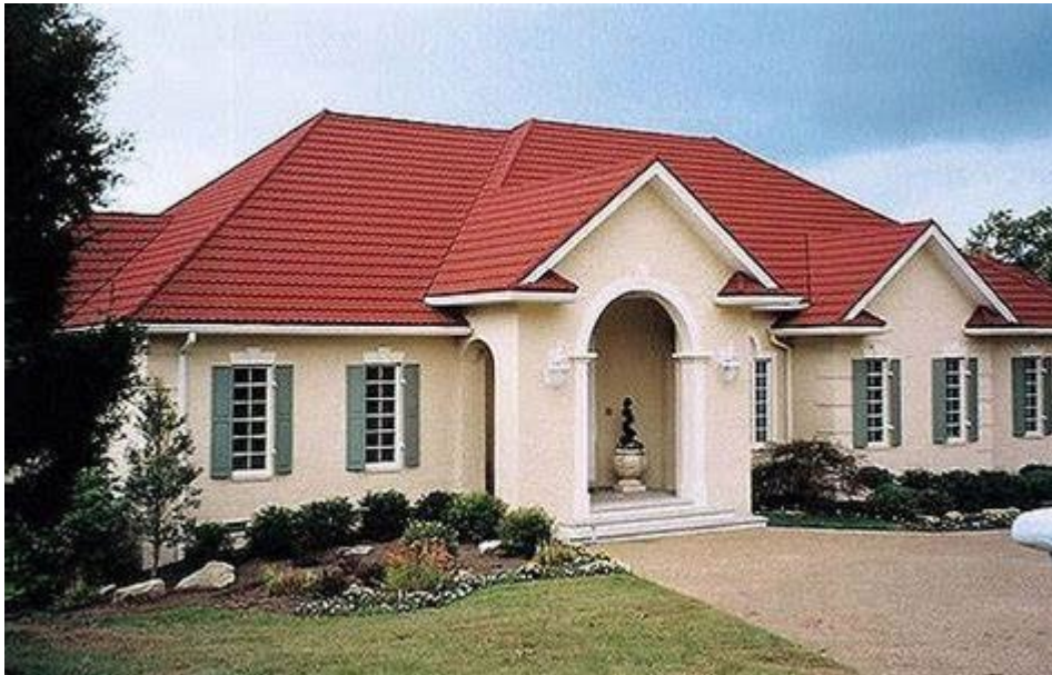
Fig 4: Low heat and energy is reflected away from roof while higher heat and energy is absorbed and convert to high heat. This roof is likely to be hot.
