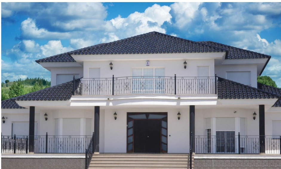
Fig 6: All heat and energy is absorbed by a black/ dark roof, almost no heat and energy is reflected away. This dark roof (and therefor the interior of the house) is likely very hot .
